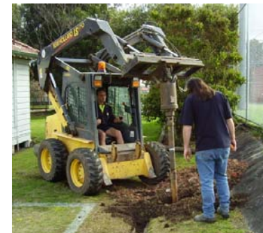
digging holes for the light poles
